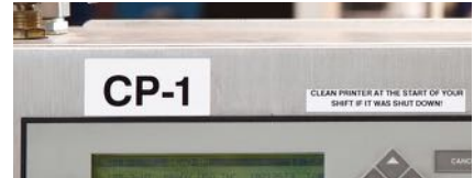
Control panel & electrical panel labels
