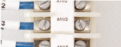
Terminal block markers
