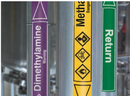
Pipe & valve marking
