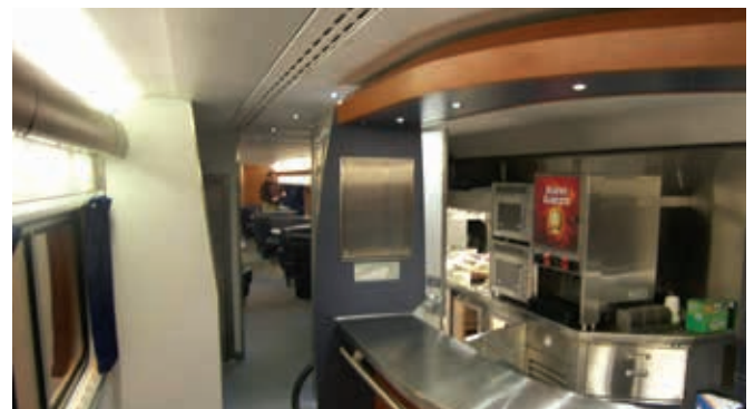
US Railroad North America Carriage LED downlight and safety lighting
