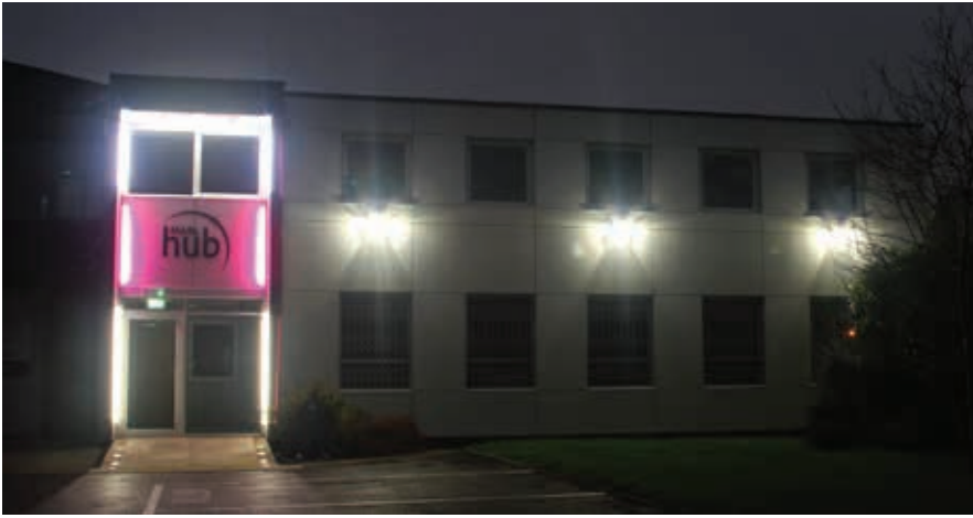
Marl Business Park, Ulverston, UK Outdoor Security Lighting & RGB feature lighting
